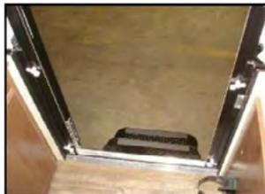
**Step 5** - The top of the door goes under the bracket that held the screen door to the ceiling. Secure the top of the door with the two dead bolts that slide over the aluminum plate (arrows).
