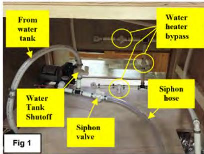
Water valves and water heater bypass
