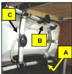
Factory installed 3-valve water heater bypass
