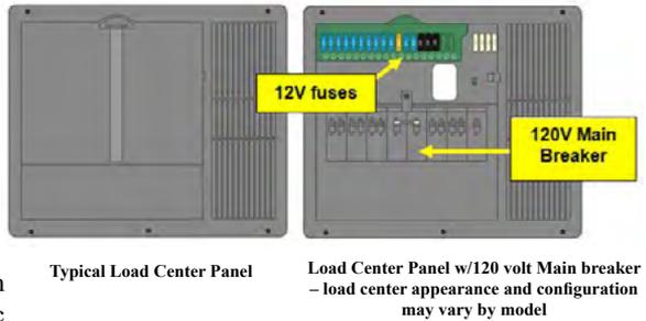
Motor homes may have separate small panels for breakers and fuses. They are normally located in close proximity to each other typically in the bed platform. The converter is also mounted separately (typically under the bed platform).
