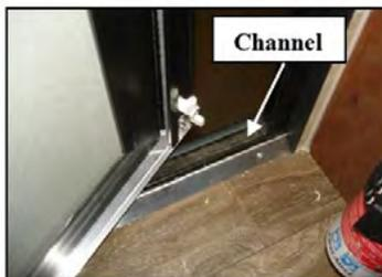
**Step 4** - Bottom of the door is in the channel, and the door frame is against the aluminum pieces on each side of the doorway. Clips turn to hold the door in place. It helps to have a second person outside to help guide the door into the channel so it is square in the frame.
